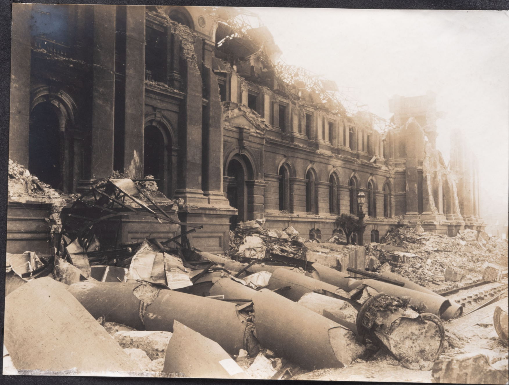
3. A study in Masonry Larkin Street wing of the City Hall.
