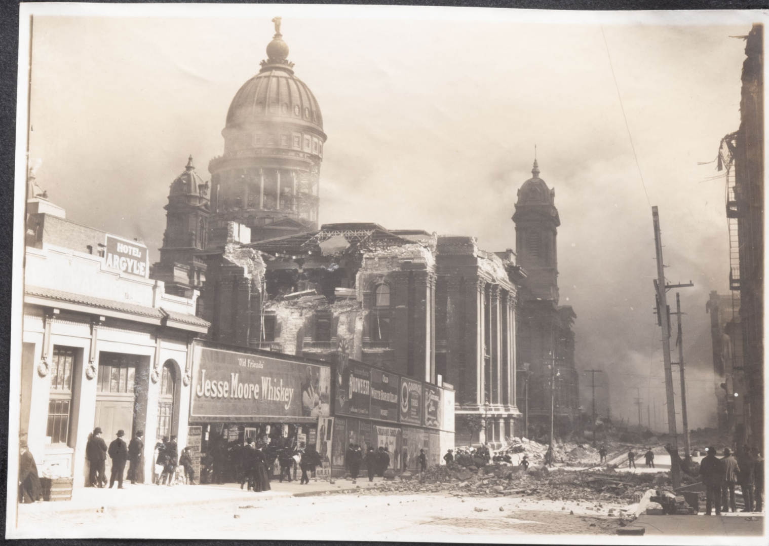
28. The fire from Hayes Valley has destroyed the Mechanics Pavilion and is now crossing Larkin St to the City Hall
