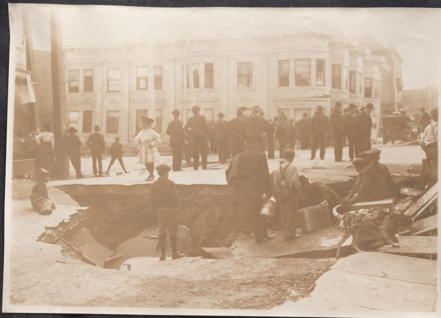
8. Valencia street break The residents obtaining water from the broken water main
