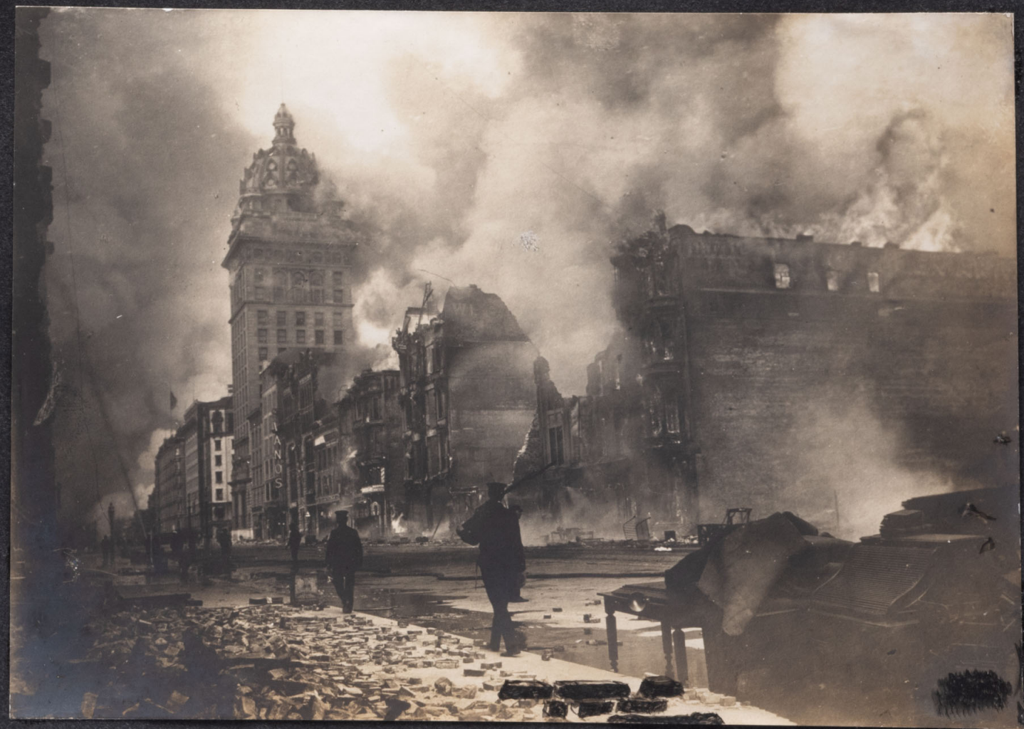
18 Fire has surrounded the "Call" Building
