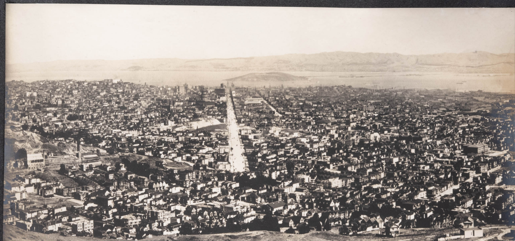
43. The same view as the preceding one, taken a few days before the fire.
