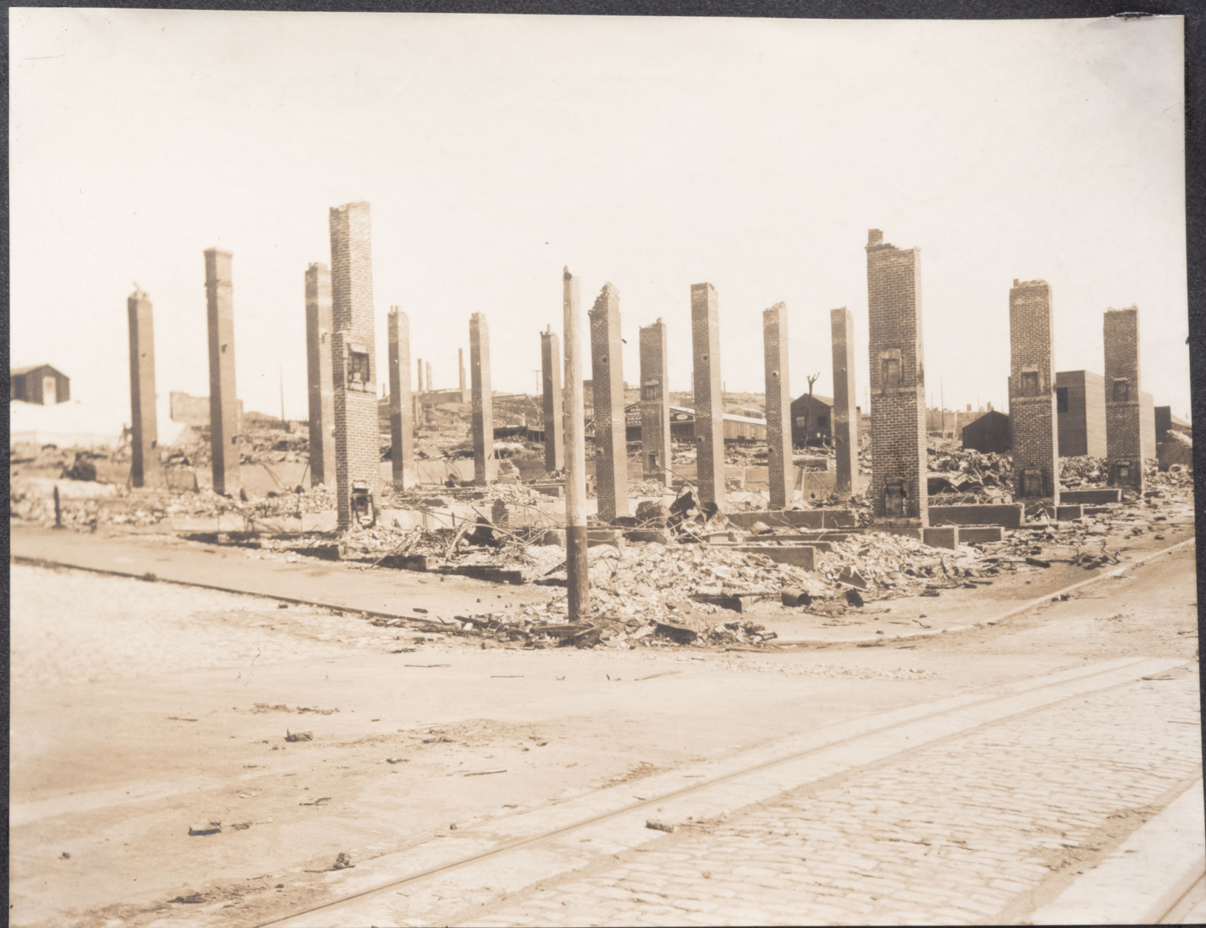
60. Forest of Chimneys, being all that remained of a large apartment house at Broadway and Hyde streets.
